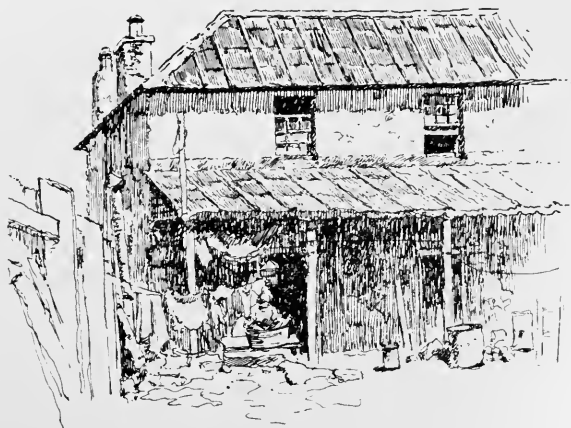
Cumberland House, Cumberland Street
